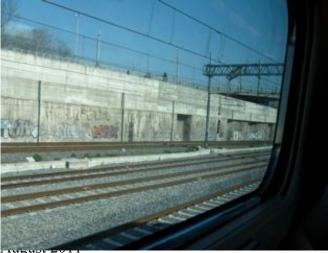
The railroad between Florence and Rome is powered by an electric overhead catenary system. It is virtually identical to Bob's electric trolley line. It is however designed for high-speed traffic. The overhead catenary wire, in the Italian rail example is almost a straight line. The wire is stretched between two supports as in Bob's boyhood example; however, it is a very shallow curve held in high tension with considerable counterweights and
